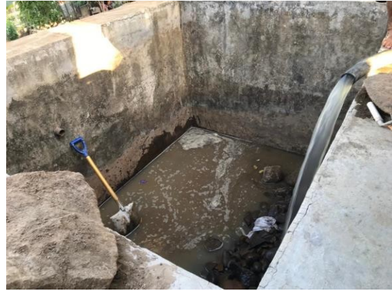
Gambar 1.4 Proses Pembersihan Bak Filter Air
