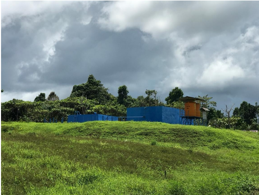
Figure 1: Water Reservoir that is not used by the Klayas Village Community (Source: Author, 2022)
